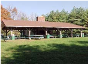
Berta Shelter (Left) at St. Patrick's County Park
