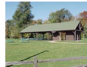
Oak Tree Shelter (Below) at Ferrettie Baugo Creek County Park
